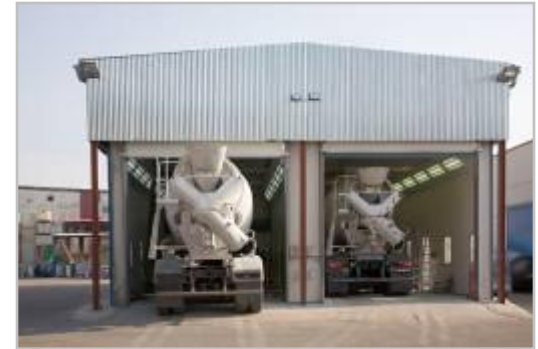
Special Cubicles where the concrete mixers can be sanded down, cleaned and have any grease removed.
